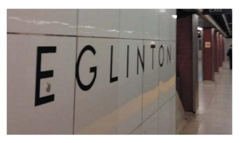
Figure 8. Original station identification signage engraved directly into Vitrolite tile panel at subway platform level.
